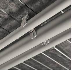
Without the need for further screws, several Basic Clips BC of different sizes can be connected by simply inserting or latching. Mounting time and costs are saved.
